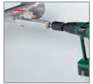
Drilling under pressure with drilling jig
